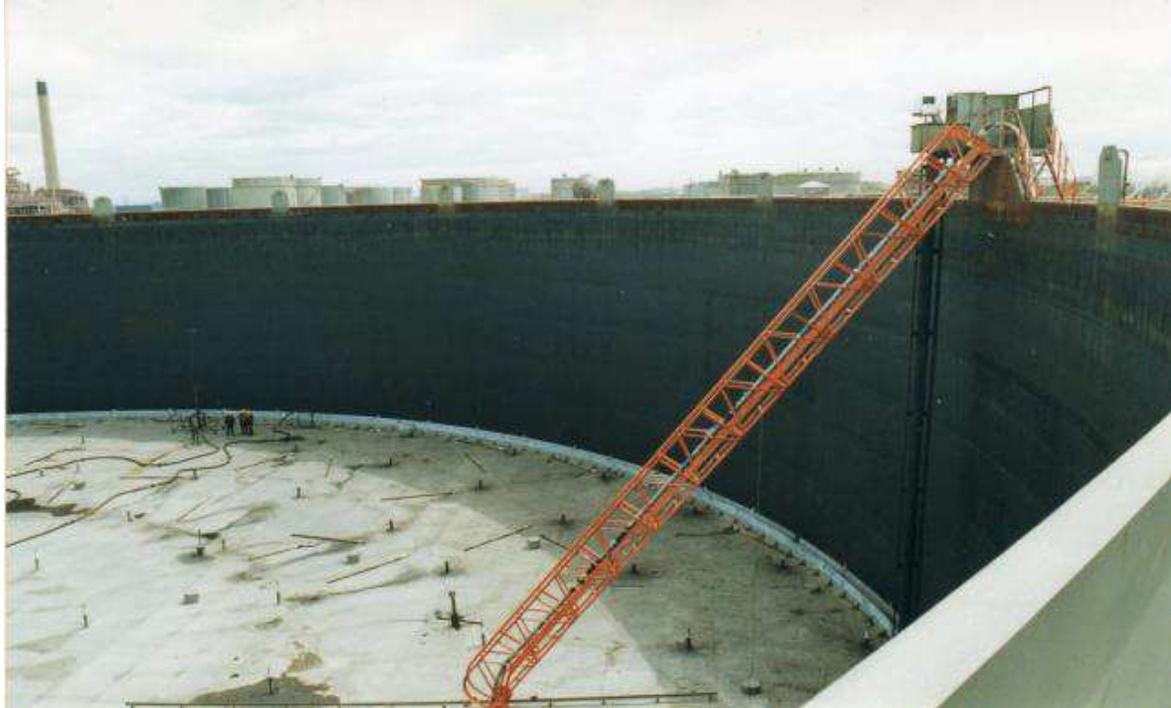
The Pump discharge hose is led up the access stairway down the roof and onto the tank roof centre
