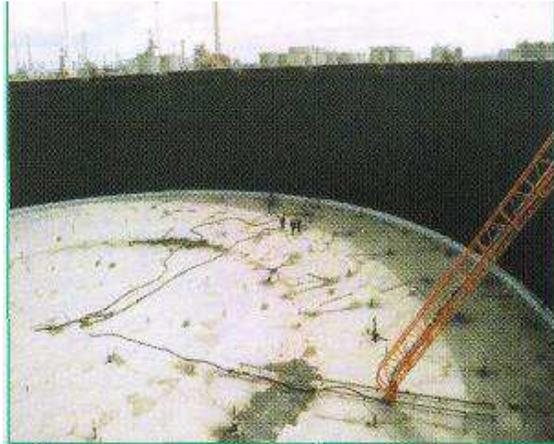
**85-meter diameter tank – Floating Roof**
